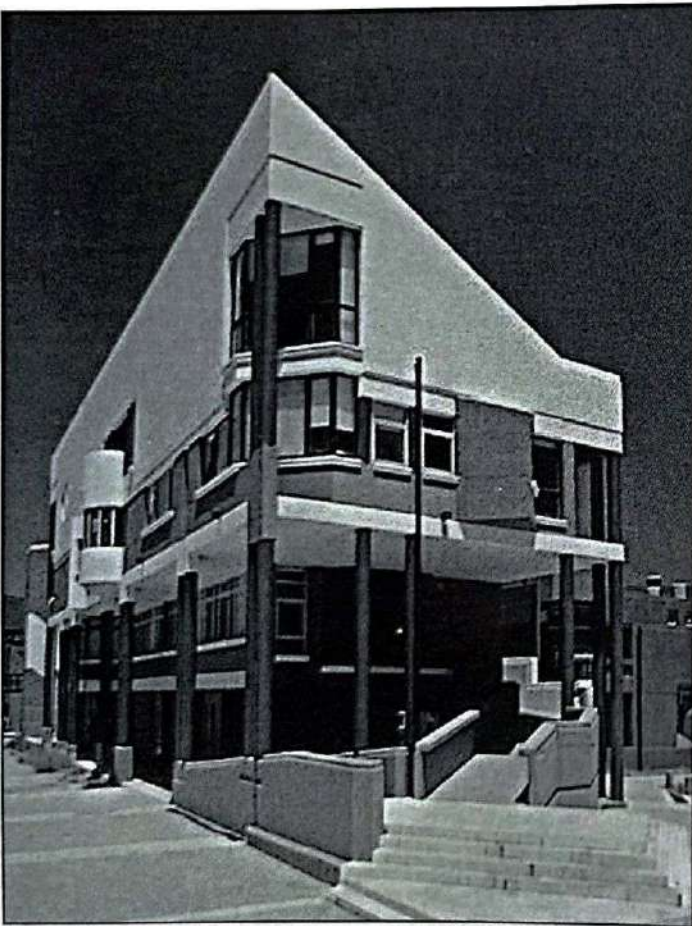
The Library of the Technical University of Crete is situated on a panoramic site, on the peninsula of Akrotiri.
